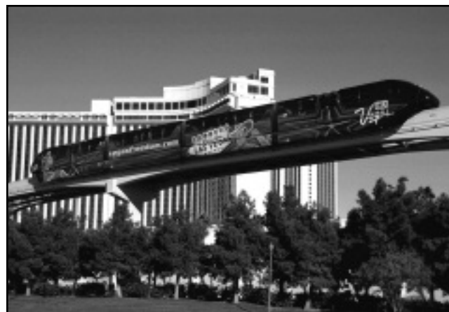
Bally’s is a station on the Las Vegas monorail, running the length of The Strip stopping at seven hotels, covering the four-mile route in 14 minutes for only $3.00.
